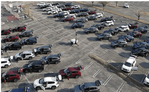
FIGURE 15 Parking lot WiFi antenna. A WiFi antenna is placed in the center of the vehicle parking lot, enabling OTA data uploads and software updates for each Raspberry Pi in each vehicle.
